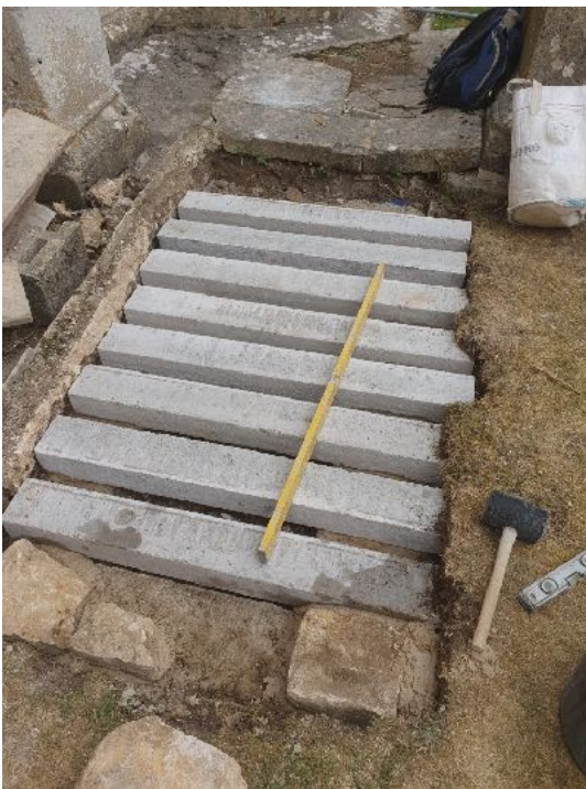
Concrete lintels set on the ring beam
