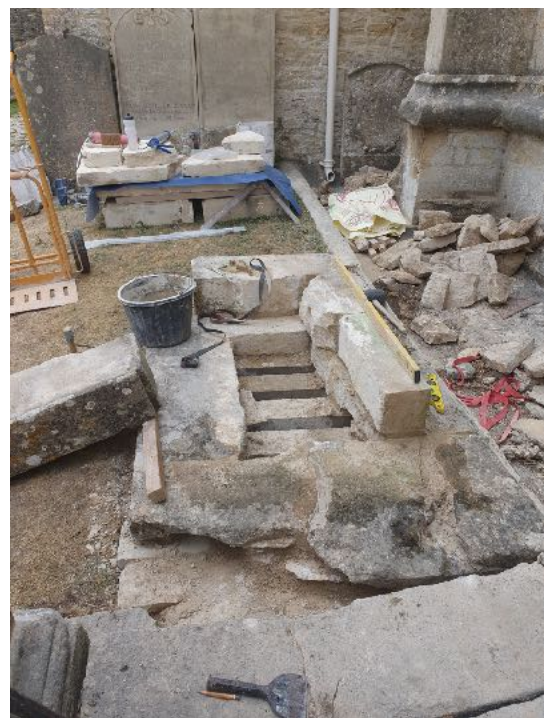
Starting to rebuild the plinth
