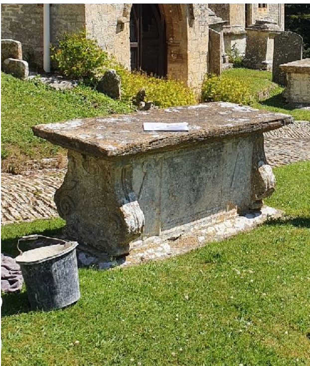
Mortar filling the spall in W lyre end
