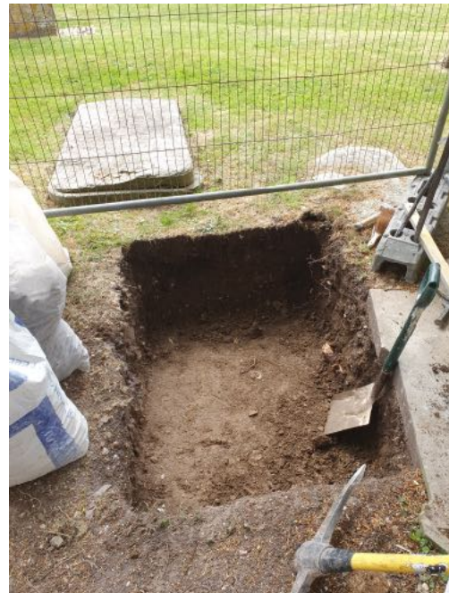
Area dug for Limecrete foundation
